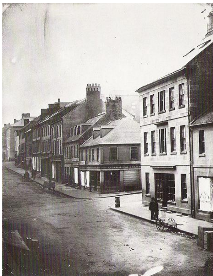
Photo: Granville Street at Duke Street, Halifax, 1854 Courtesy of Wikimedia Commons
